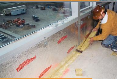
nermafiber Safing is compression fitted between FireSpan insulation and the oncrete slab edge to create a perimeter fire containment system.
